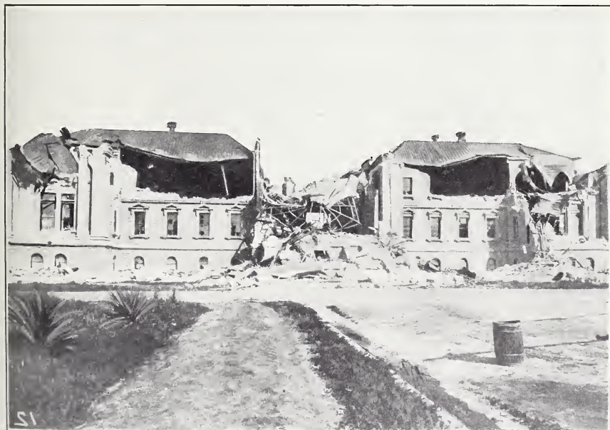
B. COLLAPSE OF BRICK WALLS, CAUSING DESTRUCTION OF STEEL SKELETON DOME OF GYMNASIUM.
